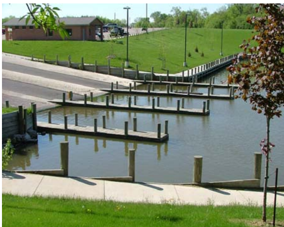
Stockbridge Harbor Boat Launch
